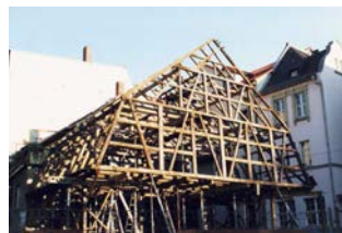
3) Messa in opera
